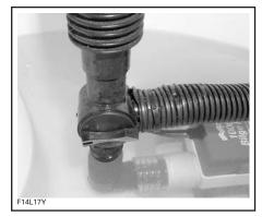
Turn fountain pump switch ON. Turn OFF when sump is drained.
