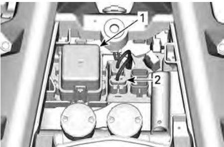
1. Front fuse box 2. DPS fuse
